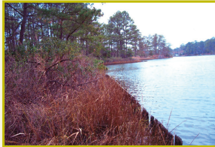
Shoreline on the Lynnhaven River with failing bulkhead (before). Photo credit: Bill Fleming
