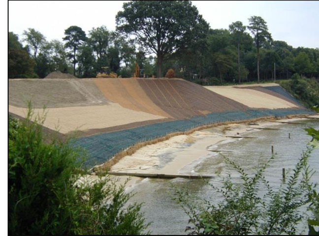
Bank Grading & Restore Riparian Buffer
